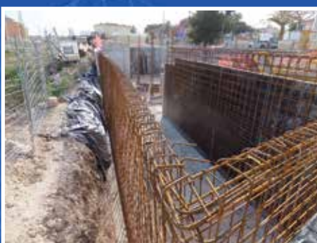
Armering gir solid grunnmur
